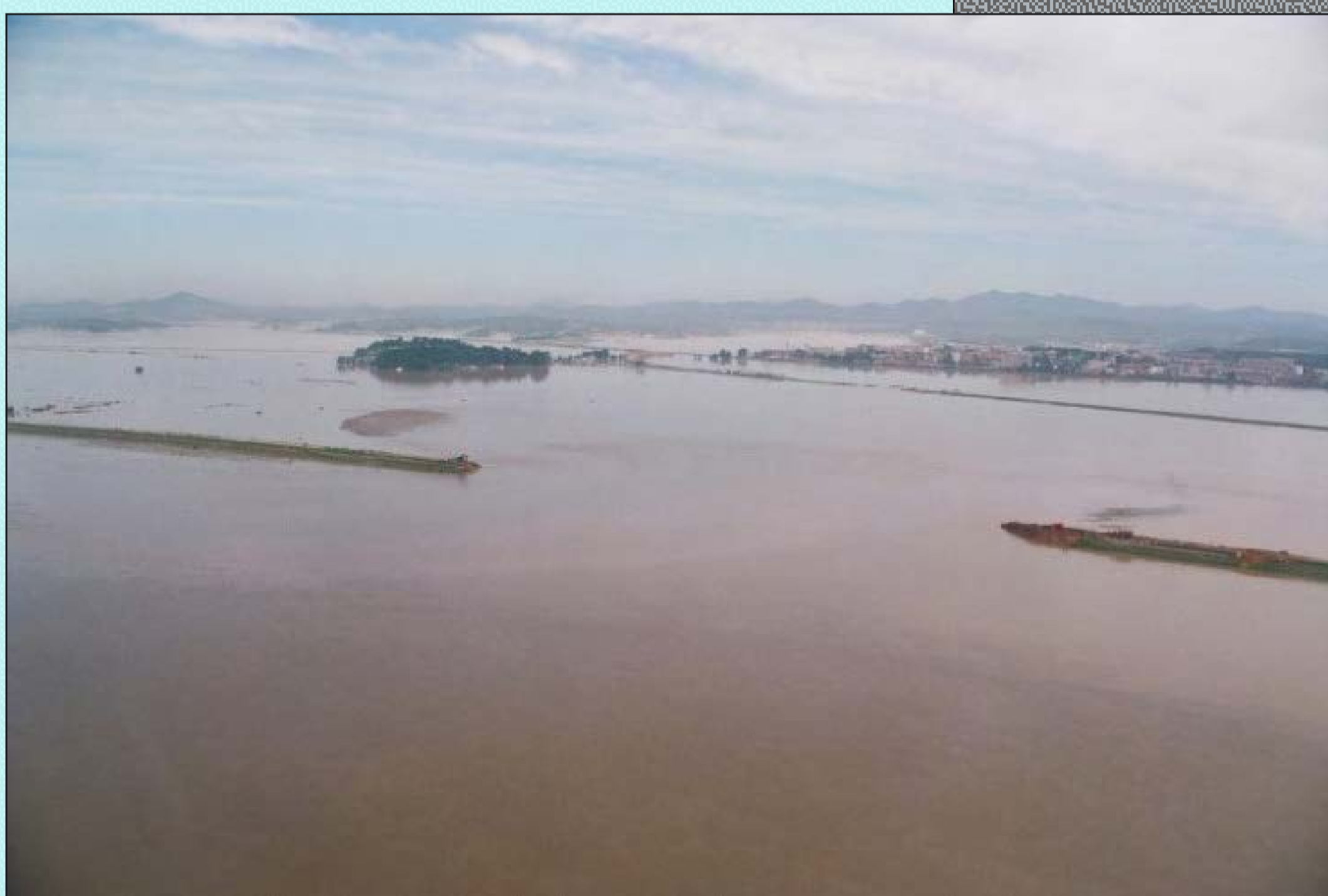
Shinpyung-ri, collapsed dam, 1990. (Image taken from the website of Goyang, accessed in 2006)
